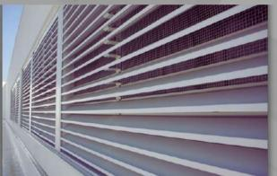
Louvers, featuring fixed or operable blades, play a key role in regulating airflow and keeping metal buildings free from dirt, water, and debris. Whether for ventilation or air exhaust, they ensure a clean, comfortable indoor environment while preserving structural integrity.
